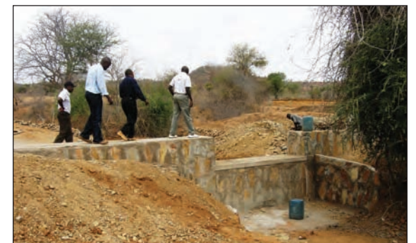
A sand dam under construction. Photo courtesy Wayne Teel
